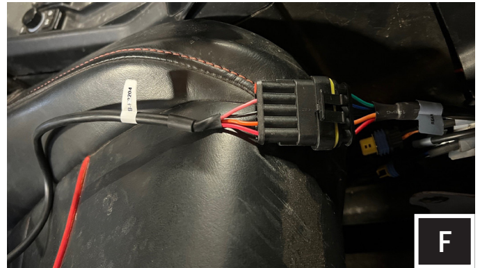
F. Run the TANGO2 rear turn signal harness (B-H3205) to the rear of the vehicle. Use zip ties to secure the cable away from any moving parts or exhaust pipes.
