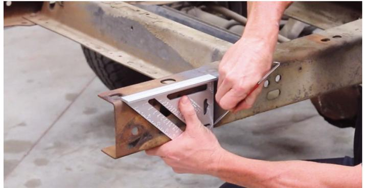
Another part of this step is fabricating an oval hole where your scribe marks are. We have routinely drilled a pair of 1/2" holes side by side and connected them using a grinder, dremmel or boring tool. As an option, you can make a single 1/2" hole aligned on center in the location of the oval scribe marks. This hole is your rear bed mounting hole and may need some amount of front to rear adjustment if you choose to make a single hole. Repeat on BOTH the DR and PA sides.
