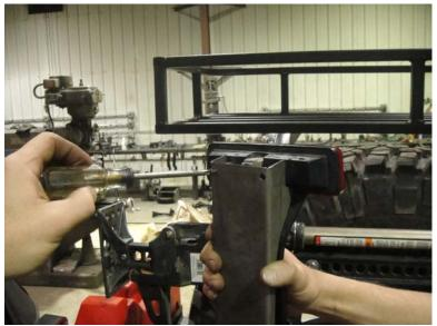
4. Screw the light into the mount. Use the screws provided with the bolt kit for the top two holes. Use the factory screws for the bottom two.
