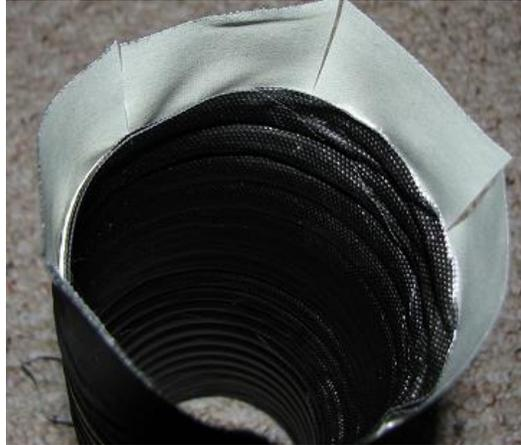
**2.30.2.** Fold over each slit pressing firmly against the hose.
