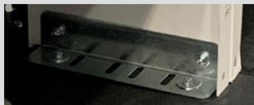
SHELF FEET ARE ATTACHED TO THE LEGEND™ EVOLVE FLOORING USING THE HARDWARE PROVIDED BY THE MANUFACTURER
