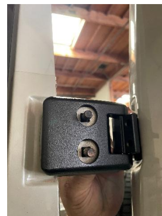
Figure 10: Upper Hinge Bolt Routing
