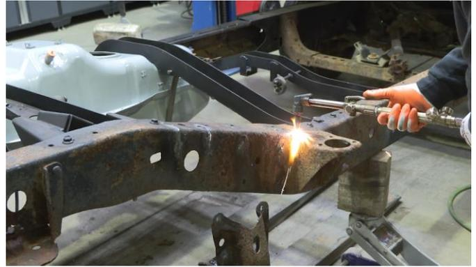
Grind away any remaining rust and debris revealing bare metal. Coat the part and work area with a weld-through primer to help prevent against further rust development.
