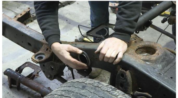
Tack weld the crossmember and shock mounts together. Then, following proper welding procedures, begin welding the part. 100% weld around all edges.
