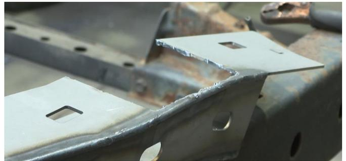
Clean the frame free of rust and debris, revealing bare metal.
