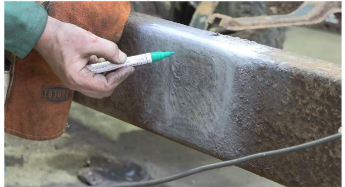
Grind the frame rail free of rust and debris, revealing bare metal.
