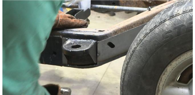
Tac-weld the part and confirm its alignment before completely welding it onto the frame.
