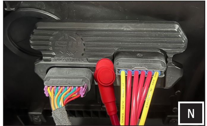
N. Slide on the rubber terminal boot (B-H3569) to the terminal post to protect from shorts.
