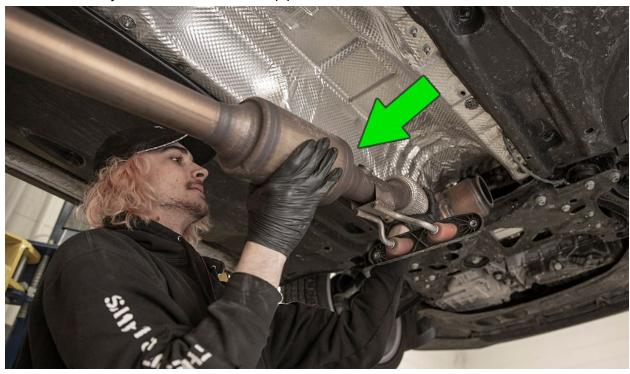
Pry the bracket off the factory downpipe then press the IE mount bracket into the factory rubber mounts. This is a tight fit and may take some force to press in.
